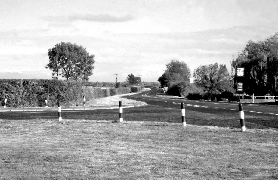
Figure 2.9 Displacement of the alignment of the Roman road (A603) as the result of medieval ploughing. This is one of three or four consecutive aratral curves, each about 200 yards long, to which the original straight alignment of the Roman road in Little Eversden was adapted during the Middle Ages by ploughmen who cultivated the fields on either side
